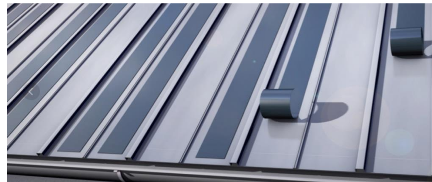
Integration of CIGS flexible modules on metal roofs ( http://sunplugged.at )
