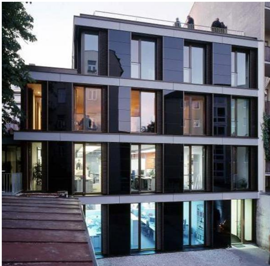
Integration of CIGS solar modules in a BIPV façade developed by Manz CIGS Technology ( www.manz.com )
