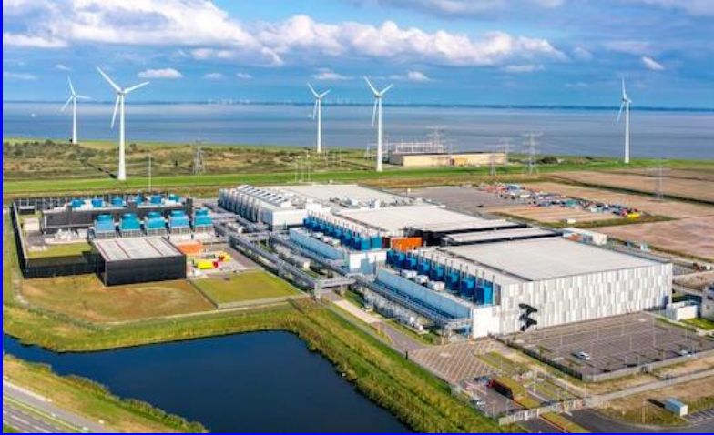
Google data centre, The Netherlands
