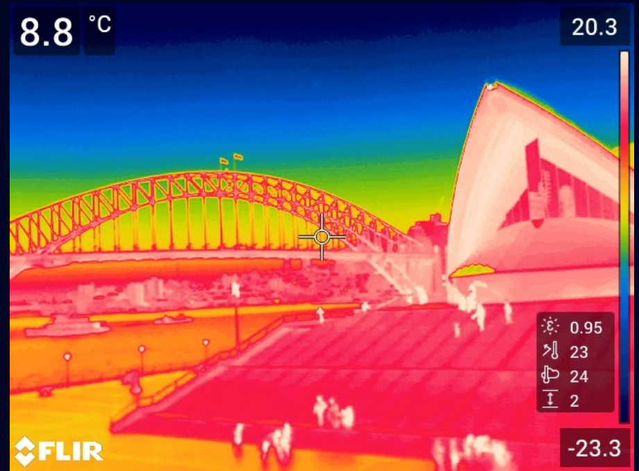
Sydney Opera House, thermal image (9pm)
