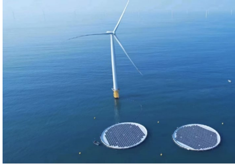
China, 500 kWp Souce: Ocean Sun
