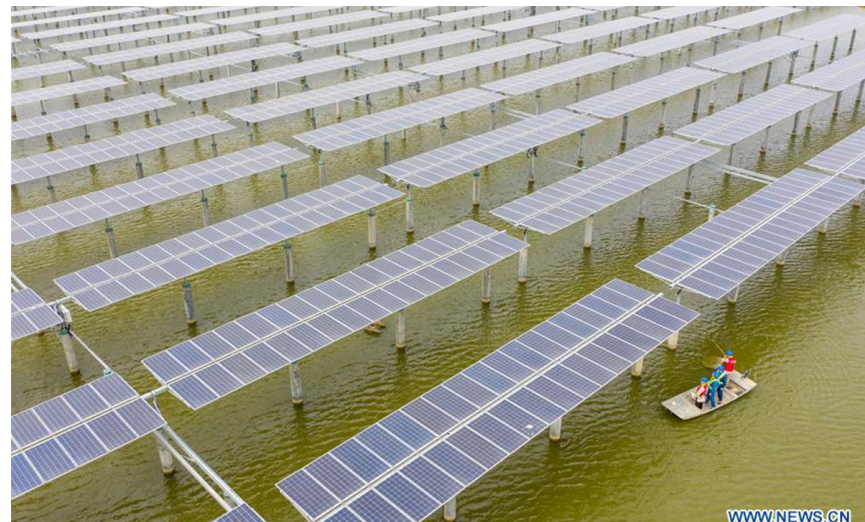
Pile/stilt-based PV
