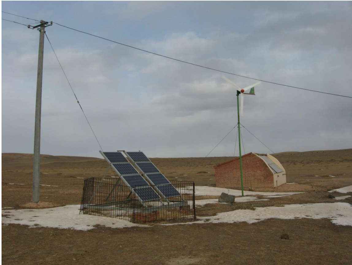
A typical solar PV / wind hybrid household system
