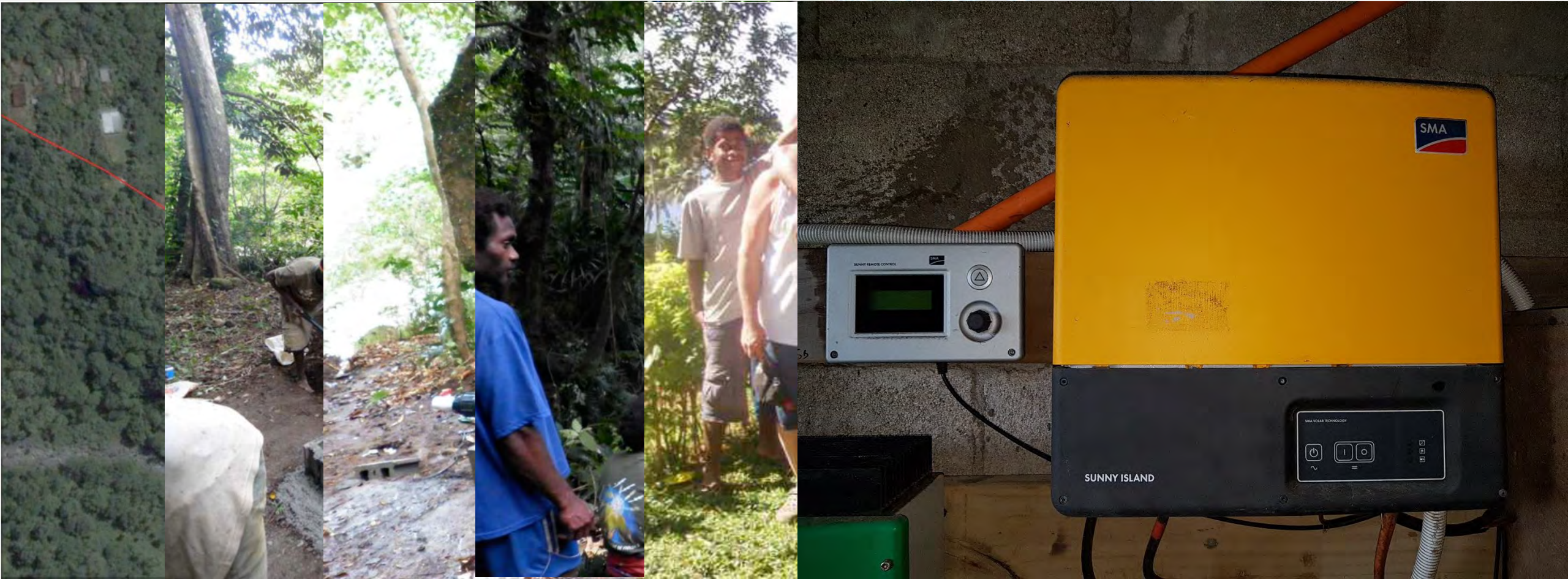
Hydro power from dedicated penstock
