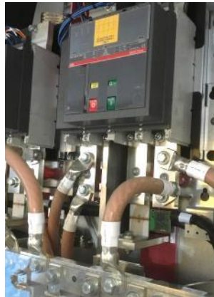
DC Load Break Switch
