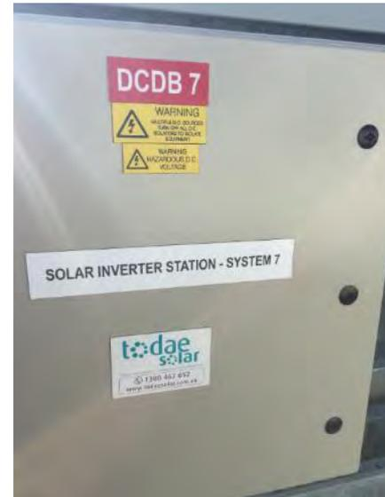
As there are 7 systems installed at one Shopping Centre premises, labelling clearly and accurately reflects which devices control which equipment.
