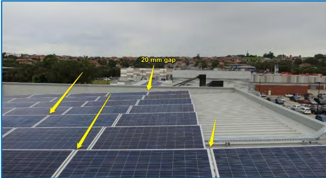
Following the guidelines from the solar panel manufacturer a 20 mm gap was left. The inclination of panels at 10 degrees contributes to better performance and less losses due to natural ventilation.
