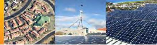
Todae Solar in partnership with Canadian Solar was selected to design, supply, construct, commission and maintain this unique photovoltaic system on a Shopping Centre with a final power of 1,217.56 kWp utilising 3992 Canadian solar panels (305Wp) and 43 SMA STP25000 inverters.
