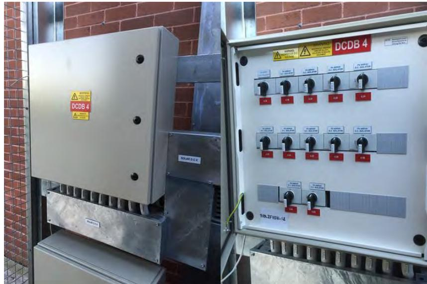
DC isolators for the inverter stations were pre-built in an enclosure, pre-wired and delivered on site so the installation team had to simply fix on the wall and connect.
