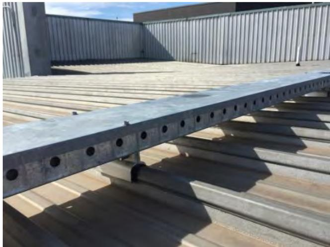
To simplify the installation while achieving best practice, the AC and DC cable trunking was carefully selected to improve the visuals, quality and performance of the system while ensuring mechanical protection.
