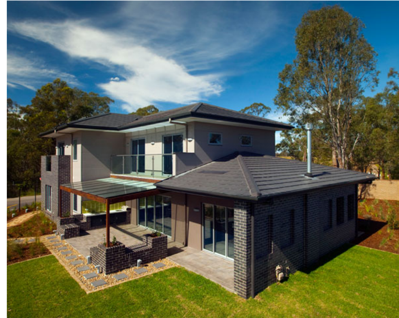
CSR house today – demonstration of how to “mainstream” an 8 star energy efficient design.
