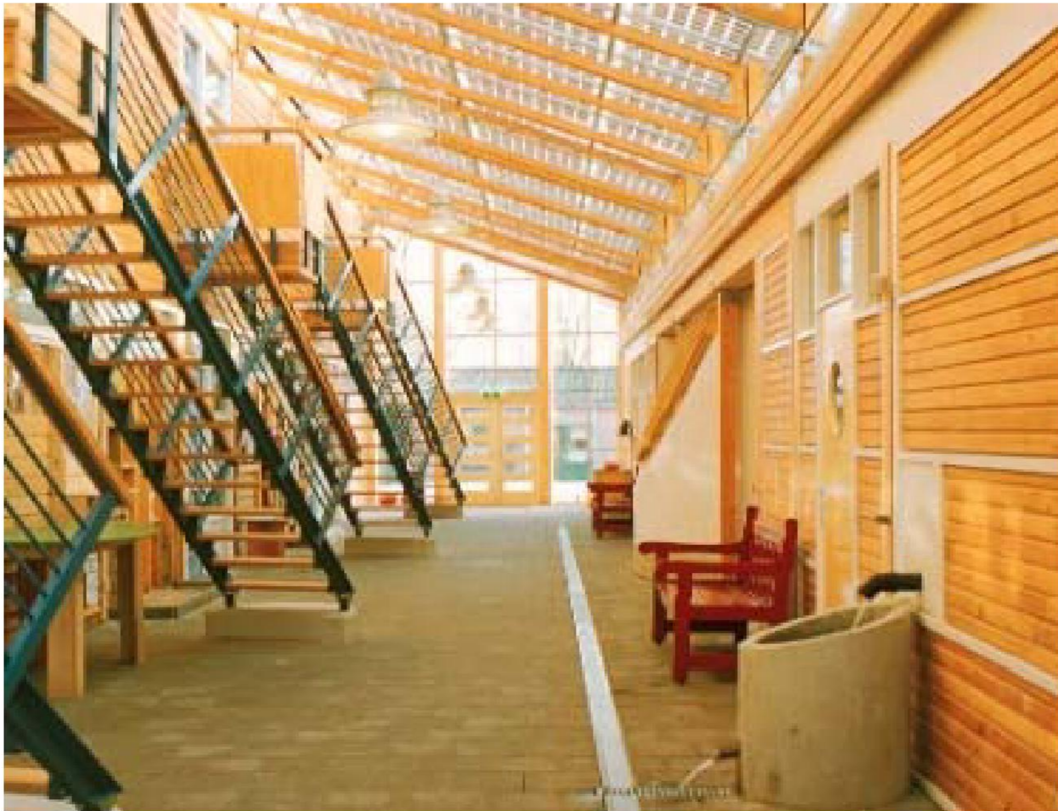
PV roof at De Kleine Aarde
